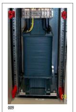
A4 Lift the transformer with the appropriate lifting equipment onto the edge of the mounting plate and push the transformer all the way into the cabinet. (see picture 009)
