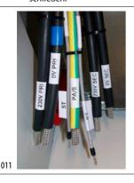
Systems  $\leq$  8 kVA max. 1.8 Nm Systems > 8 kVA max. 3.7 Nm Terminals "ST" max. 1.5 Nm
